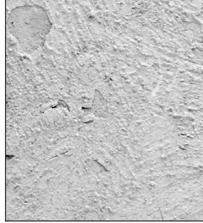
Sand the peeled areas of the lid and reapply the coating.
